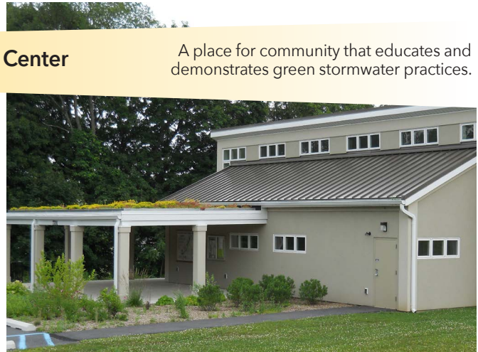
The Welcome Center's green roof helps to capture rainwater.
