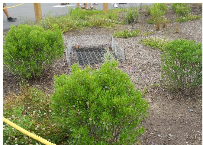
Rain gardens help to absorb and filter stormwater runoff from the parking lot.
