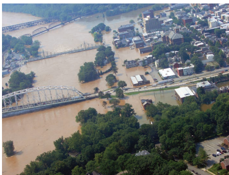
Flooding at the confluence of the Lehigh and Delaware Rivers in 2006. Photo courtesy of Frank Chisesi
