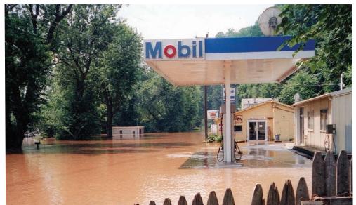
Flooding along Route 611 north of Easton (2006). Photo courtesy of Patty Caffrey.
